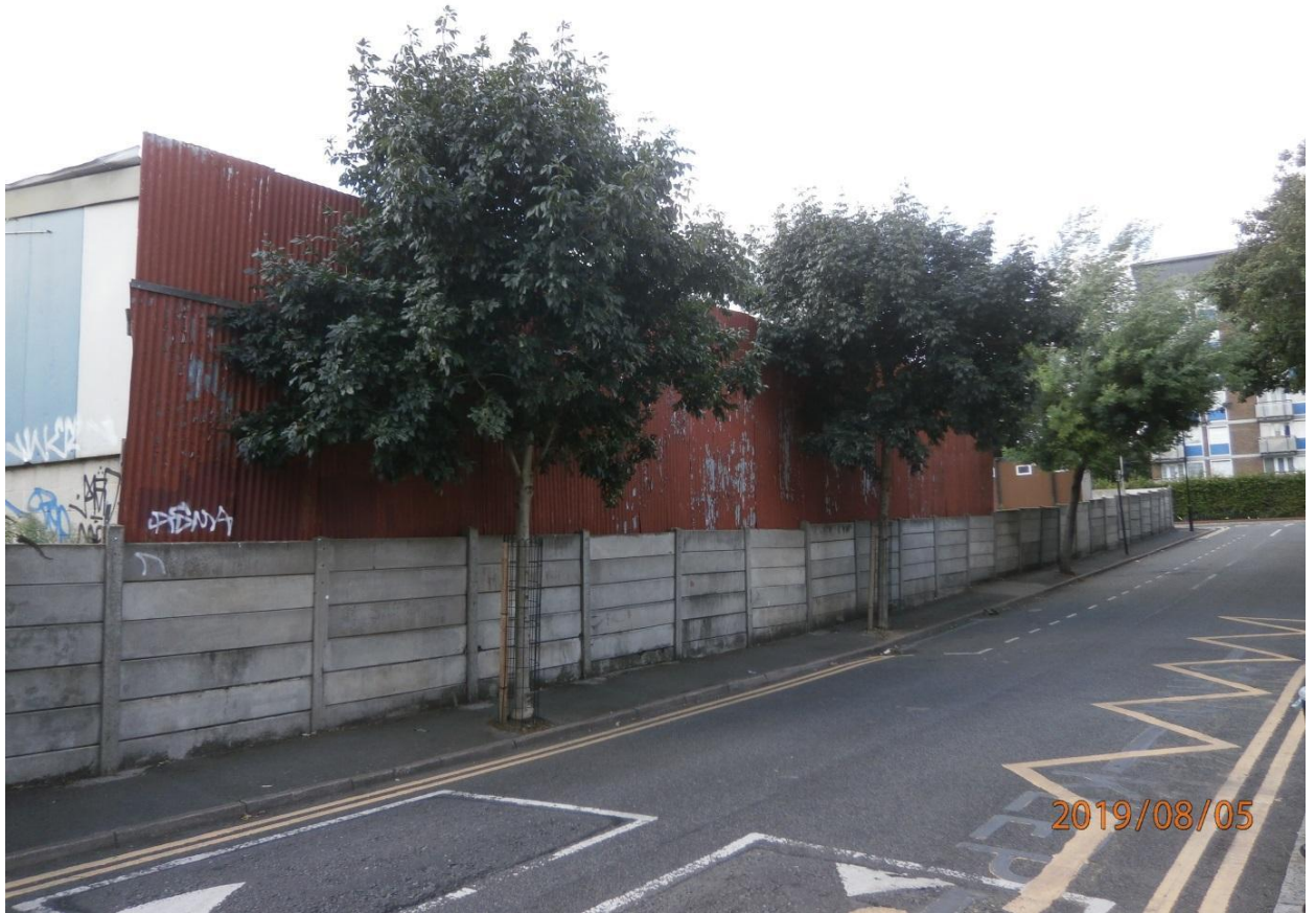
Two storey warehouse along Pearson Street:
